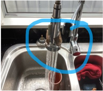
Damaged tap. Recommend repair
