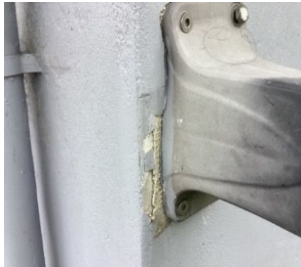
Blocks not sealed correctly. Recommend to repair and seal.
