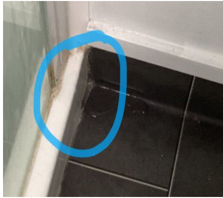
Shower is leaking in corner.
