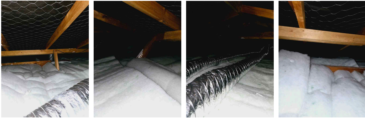
Ceiling Insulation Photos
