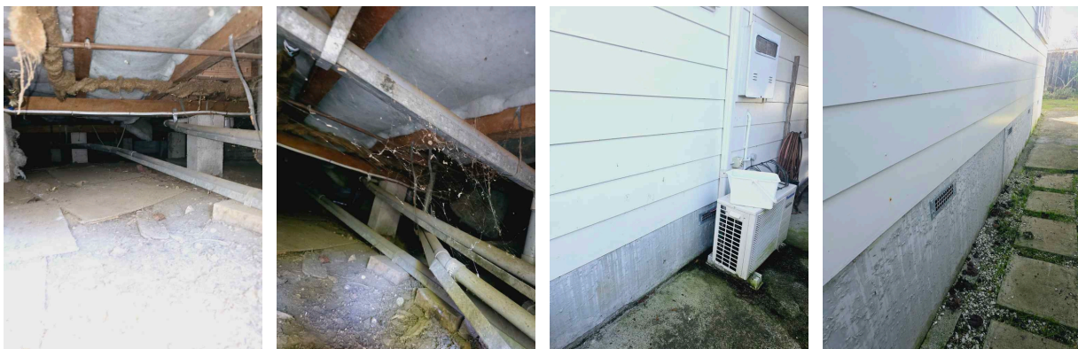
On-Ground Vapour Barrier Photos
