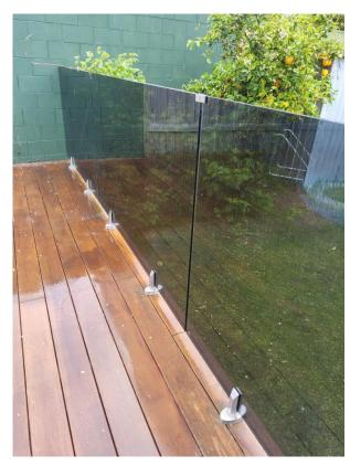
All materials / components are durable and erected so as to inhibit any child less than 6 years from climbing over or crawling under the fence from the outside  Complies with Fencing of Swimming Pools Act 1987
