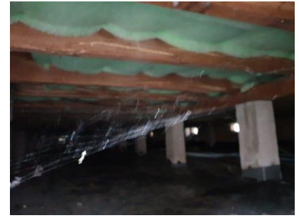
Insulation & Moisture Barrier
